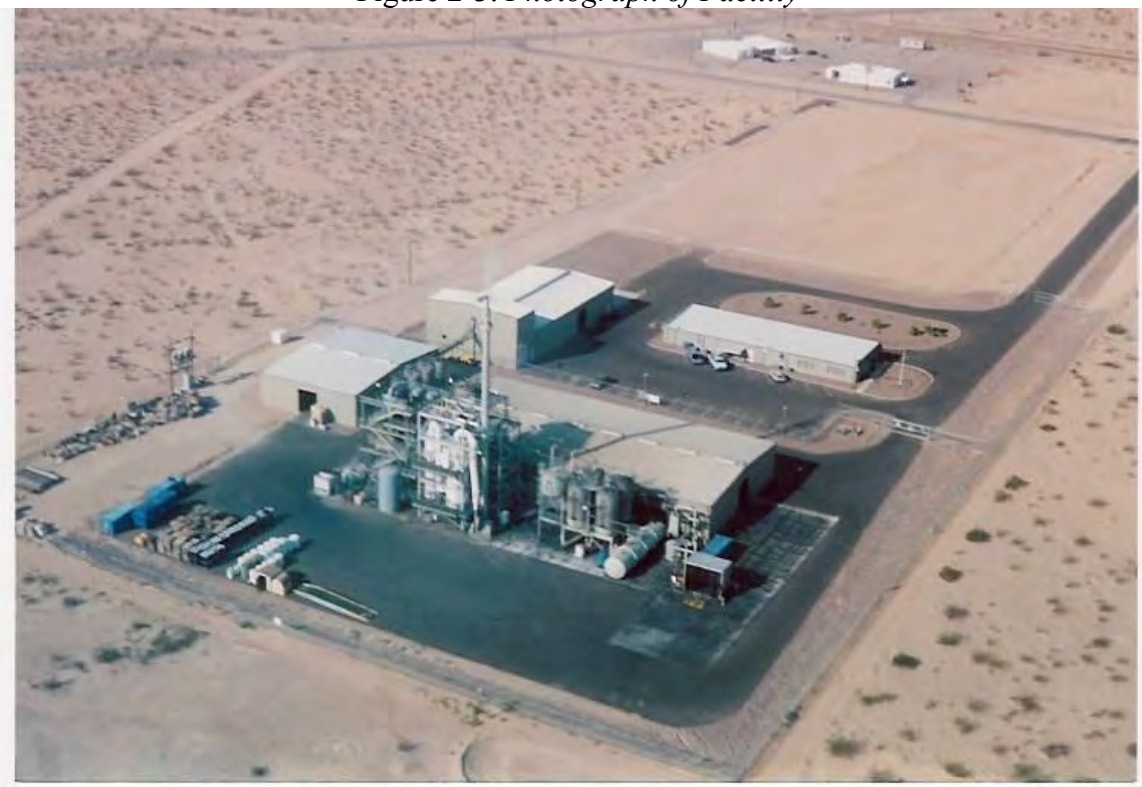
Figure 2-3. Photograph of Facility
